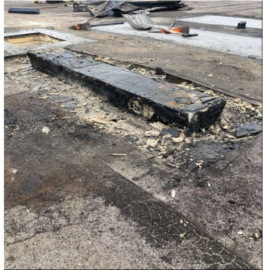
Roof curb removal has begun
